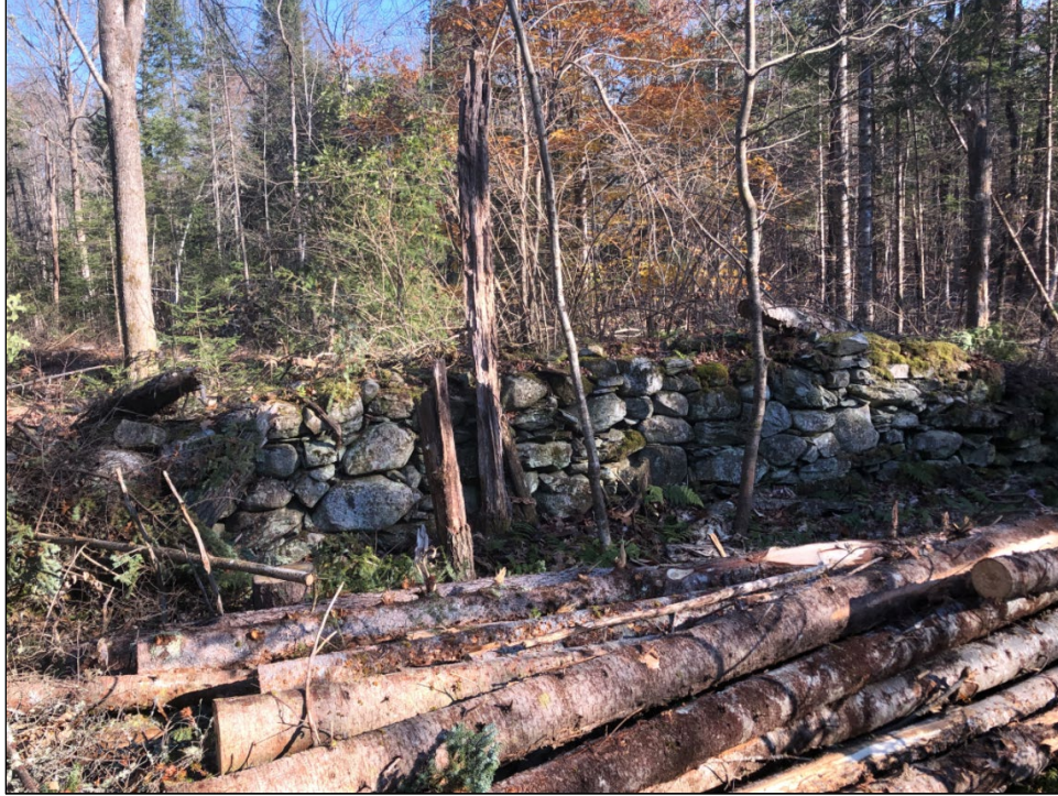
Figure 5-58. Intact southern wall of structure at Site MP-1, facing northeast.
