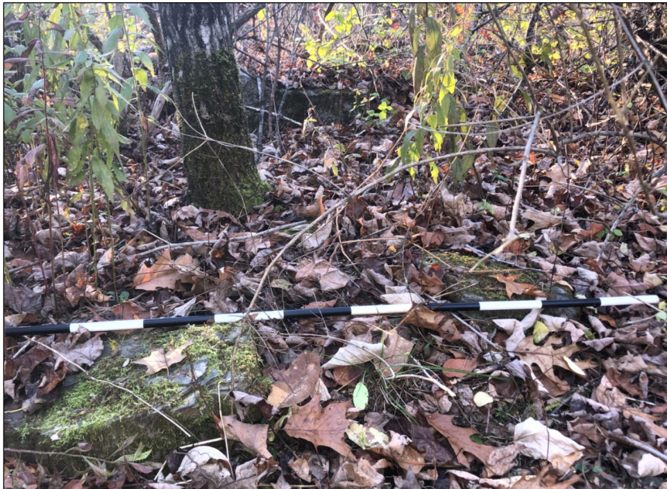
Figure 5-16. Slab footer at Site MP-15, facing west.
