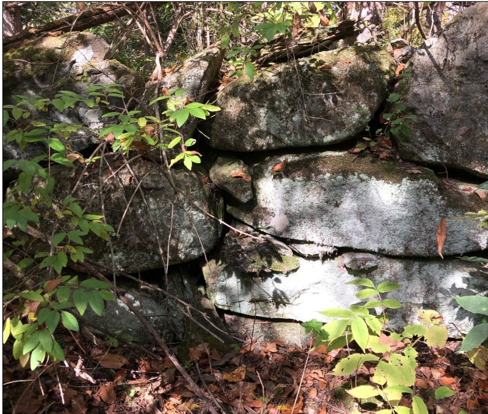
Figure 5-25. North wall of the Site F-2 foundation, facing north.
