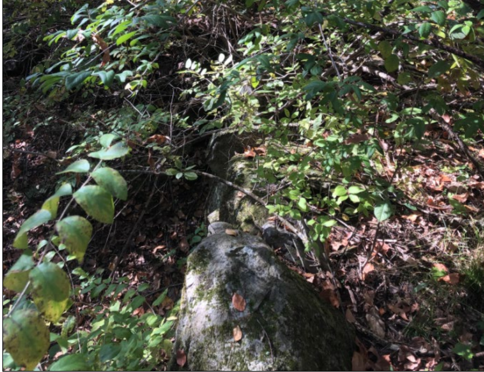
Figure 5-26. View from northeast corner of Site F-2 foundation, facing west.
